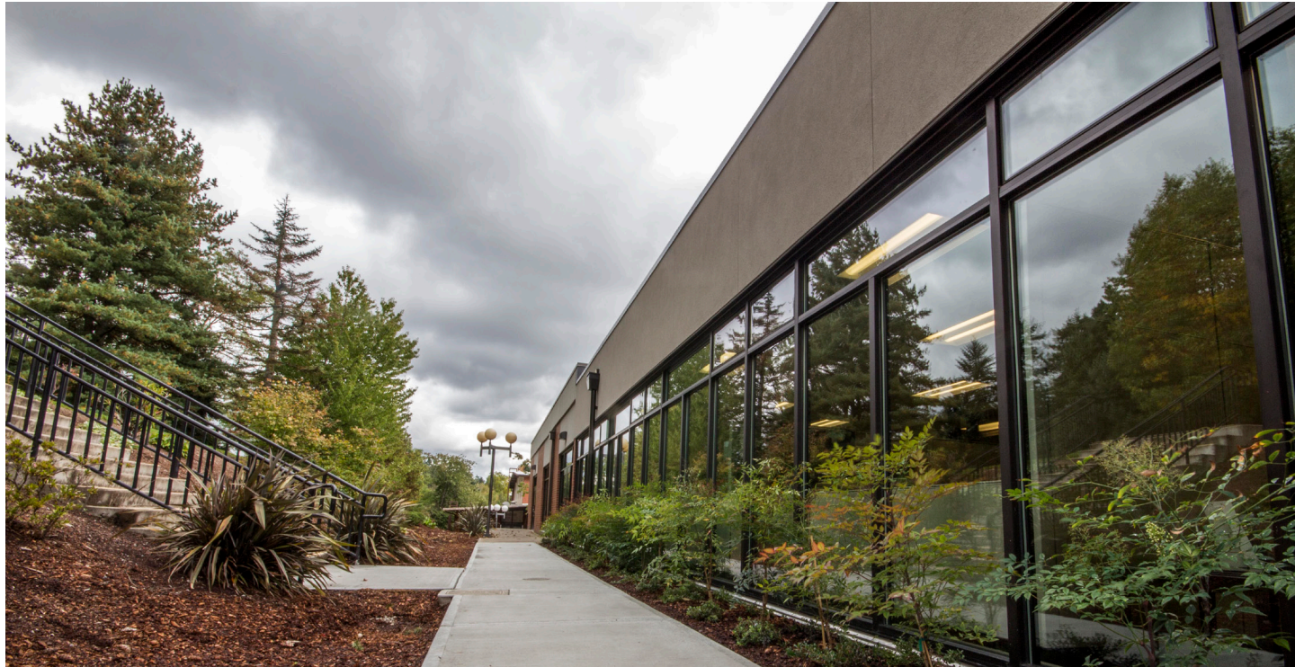
New offices extend over the three additional classrooms in Egtvedt Hall, expanded during summer 2013. Story photos by Tim Jackson.
